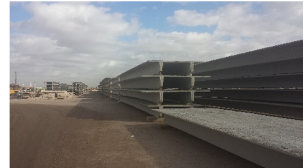
Set Prestressed Concrete Members at TPAC (Alqattan, 2013)
